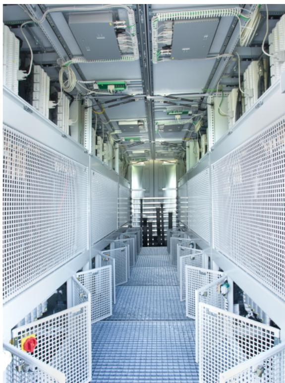
9 MW multi-level, high voltage converter
